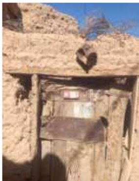
Picture 17 : Wood damage to doors
